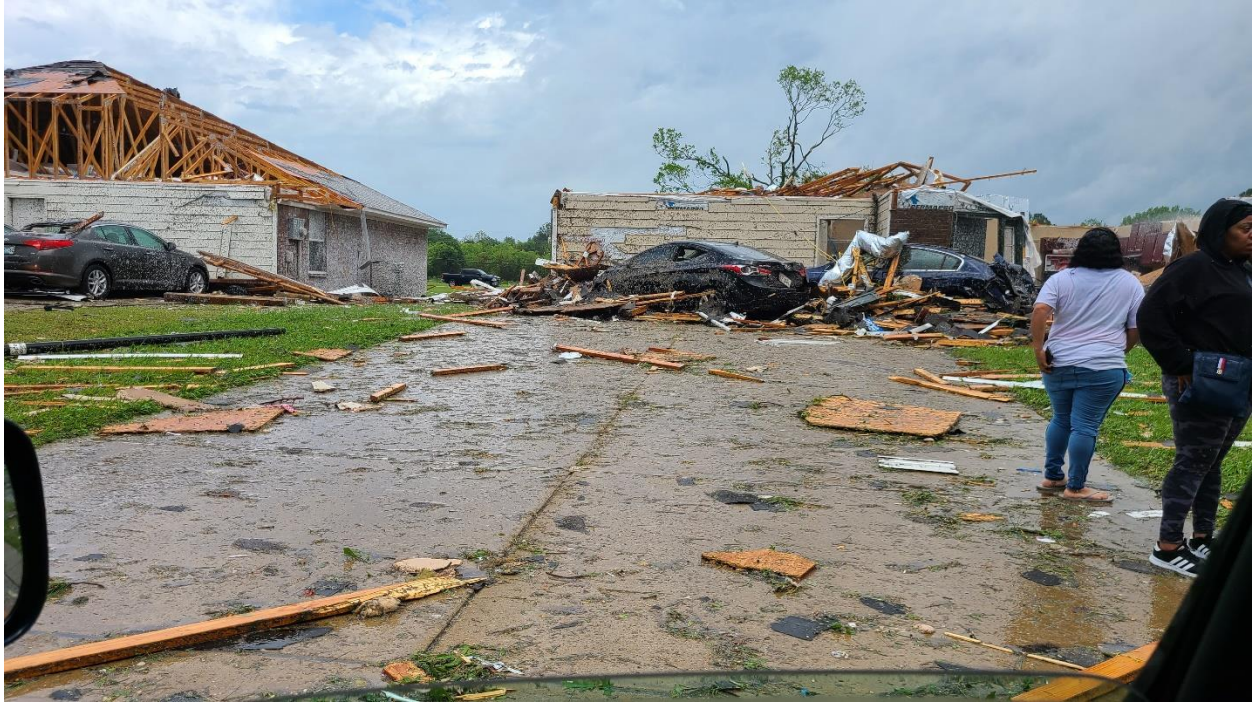
Figure 8 EF3 Damage in Monroe Subdivision. Photo by Keith Brooks
